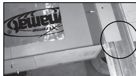
Use 1 \frac{1}{2} " side of metal angle for solid mount on hat channel
