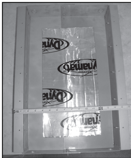
Back box with 1 \frac{1}{2} " angles for hat channel attached
