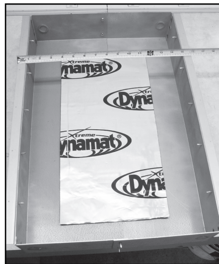
Back box with \frac{3}{4} " angles for metal studs attached
